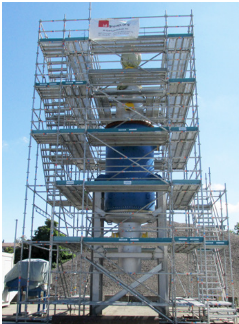
Educator Anlage in Zofingen
