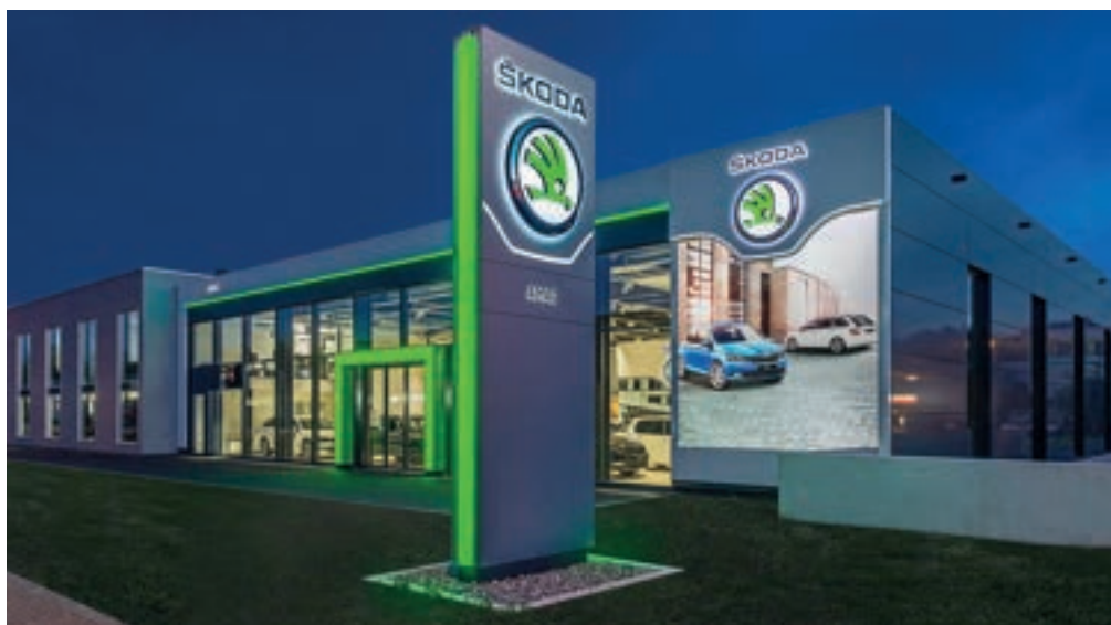
Neubau AMAG Solothurn in Zuchwil
