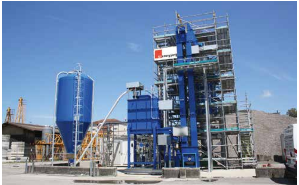
TCC Educator Anlage in Zofingen
